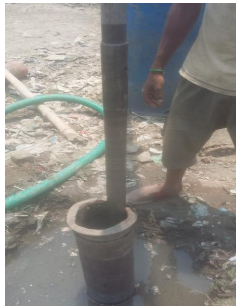
Figure 5 Soil sampling for Geotechnical and Topographical Survey at Mollar Bheri
